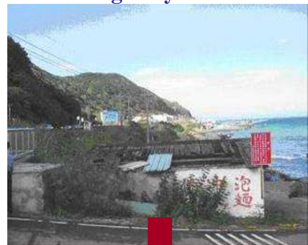
Removal of Illegal Structures on Provincial Highway No. 2
