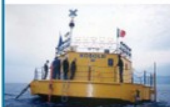
Enermar system Sea testing in the Strait of Messina, Italy (Ponte di Archimede, Italy)
